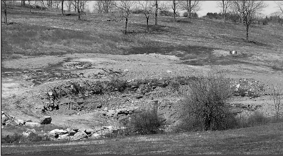
Figure 2. An example of a cave entrance excavated using a trackhoe. This site is adjacent to an industrial park that overlies most of the cave. It will take a few years for the entrance zone area to regain a pre-dig condition, but it was felt that the benefits of gaining access to the cave for environmental monitoring and resource inventory outweighed the disturbance caused by employing heavy equipment at this far from pristine site. Photo by W.K. Jones.
