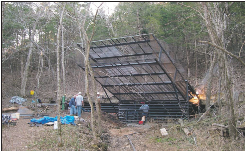
Chute Gate with a supporting Bay Window, Tumbling Creek Cave, Missouri. Photo by Bill Elliott.
