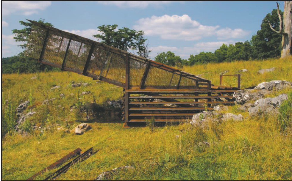
Chute Gate on a Cupola, Grigsby Cave, Virginia. Photo by Jerry Fant.
