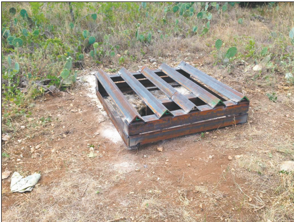
Flat Gate raised slightly for critter access, Bering Sink Cave, Texas. Photo by Jim Kennedy.
