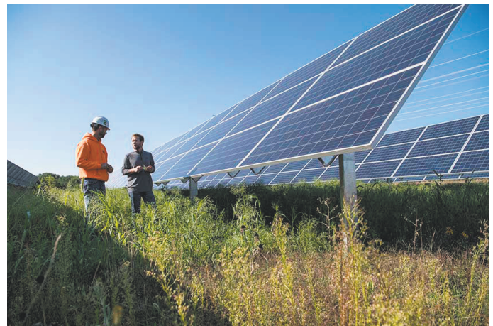
Figure 3. A well-planned solar site which has been revegetated with native plants provides the best natural filtration for storm-water and provides a high level of protection to the karst resource.
