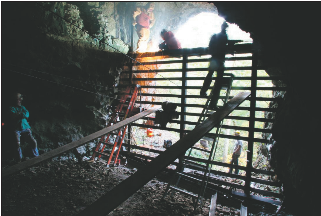
Half Gate (in Progress), Bat Cave, Oregon County, Missouri. Photo by Jim Kennedy.
