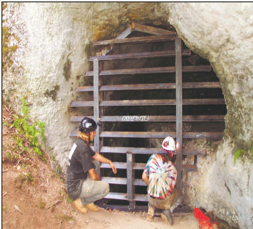
Basic Cave Gate, Lower Entrance to Bacon Cave, Virginia. Photo by Jim Kennedy.
