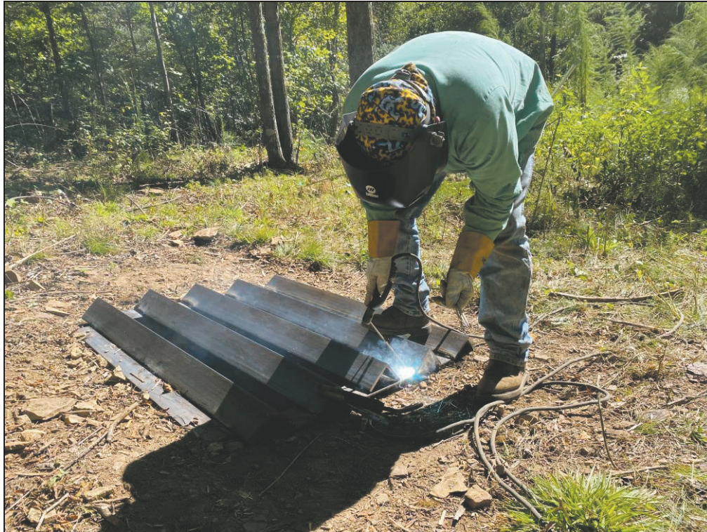
Flat Gate under construction, Weaver Cave, Alabama. Photo by Jim Kennedy.
