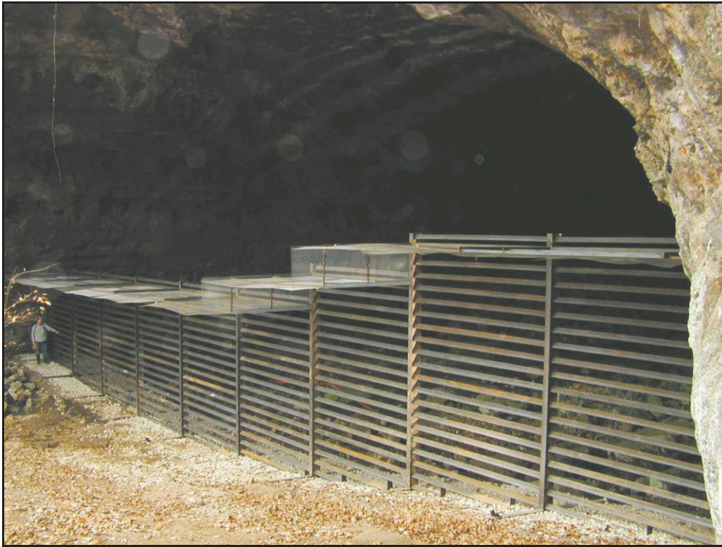
Half Gate, stepped to match the ground contour, Great Spirit Cave, Missouri. Photo by Bill Elliott.
