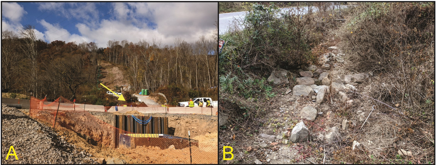
Figure 5. Doe Creek Crossing (Direct bore). A. Looking down 70m long path of bore, arrow indicates channel. B. Dry stream channel of Doe Creek with quartzite cobbles, ~ 3 m wide.
