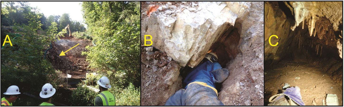
Figure 2. Small cave in pipeline trench, August 2022. A - location of cave in trench on slope; B - cave entrance; C - full extent (15 feet) of cave, now destroyed.
