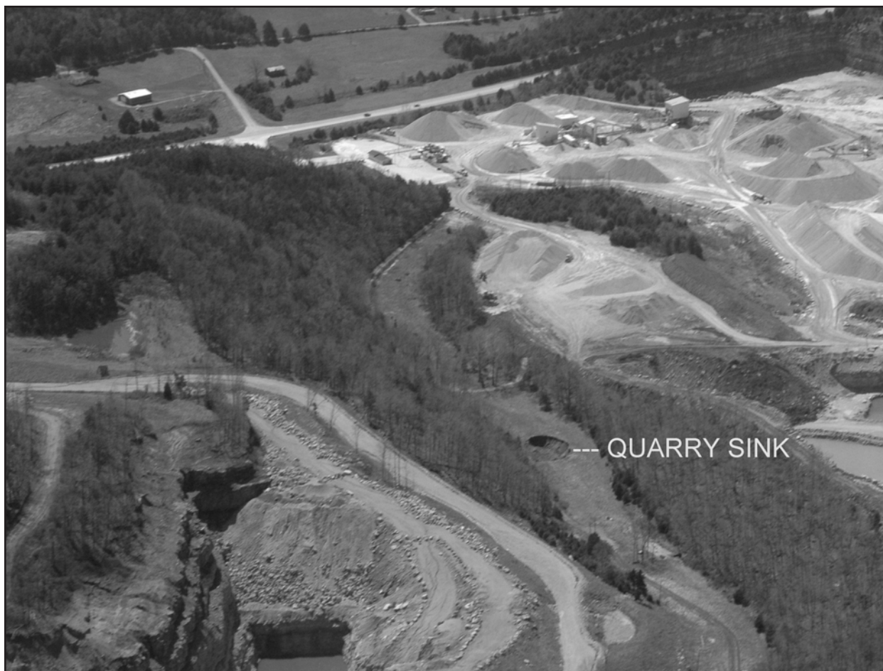
Figure 2. Kentucky Highway 80 crosses over the Sinking Valley Cave System just south of the collapse feature known as Quarry Sink.
