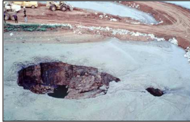
Figure 3 This post-collapse view of the West Plains Lagoon shows two sinkholes that developed as the lagoon drained.
