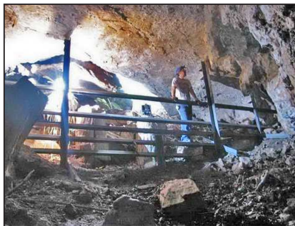
Figure 9 A cave gate under construction on a hibernation cave.
