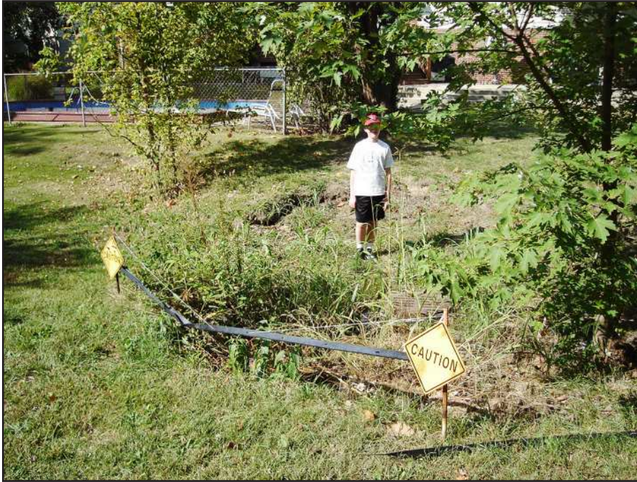
Figure 3. Collapse near a storm drain situated in a sinkhole in the Concord area. The capacity of the natural bedrock conduits is too small to drain storm water as fast as it is delivered, so this yard frequently floods to depths of several feet (Stop 3).
