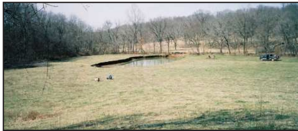
Figure 8B Berg Sink, second week of March 2005. The collapse had developed to a water-filled "spring" and had dimensions of 76 by 30 m (250 by 100 ft.).
