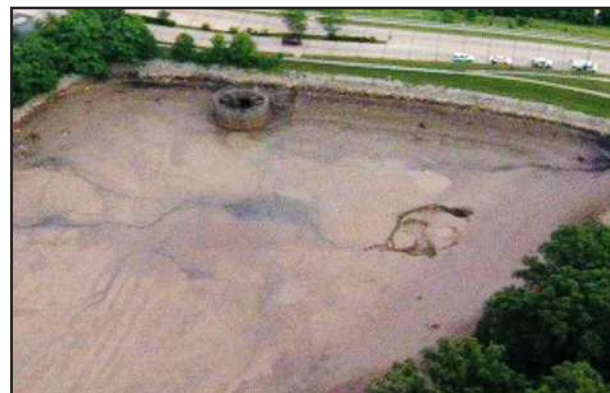
Figure 6B Post-collapse aerial view of Lake Chesterfield showing sinks that formed at the cave beneath the lake.
